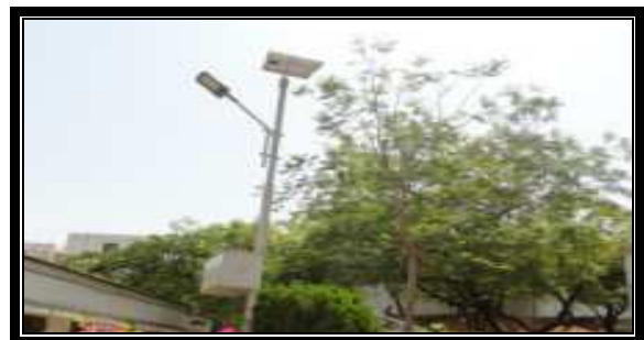
One of the Solar Light installed in MJCET
